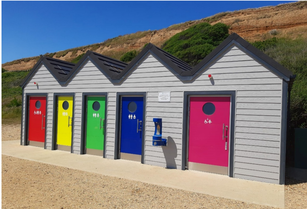
Barton Beach Public Toilets
